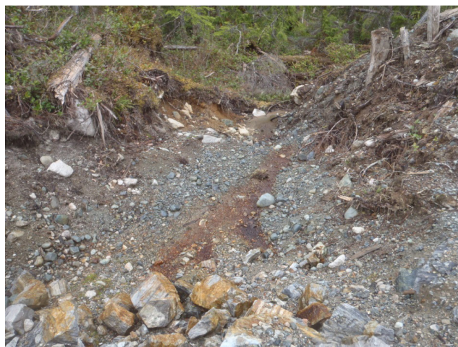
Figure 1. Iron staining downstream from a culvert outfall resulting from acid rock drainage generated by road ballast. Unrecognized use of acid-generating rock adjacent to streams can cause local pH levels to drop below 4.0 and make the heavy metals associated with sulphide deposits more dissolvable. While acid road drainage is not in the same league as acid mine drainage, impacts can be severe on local fish, plants and wildlife.
