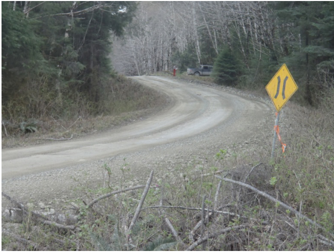
Figure 1. While this road next to a stream on northern Vancouver Island is built with potential acid-generating rock, it does not seriously impact water quality. The FREP WQEE value at this site was determined to be “very low” for fine sediment generation, which also applies to acid-generating discharge. All road (and ditch) drainage is designed to flow away from the bridge and be deposited on the forest floor away from the stream where it can be neutralized. Forest floors have a very high buffering capacity for acid rock drainage.
