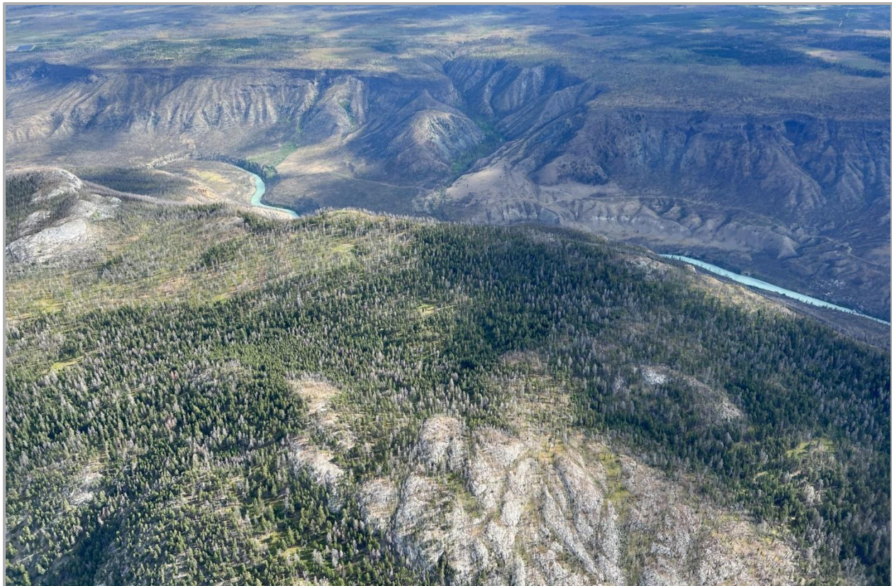
Fire damage and old Douglas-fir beetle damage SE of Hanceville, looking north toward the Chilcotin River
