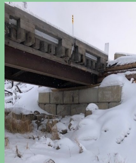
At TSN an engineered bridge has been installed over a watercourse.
