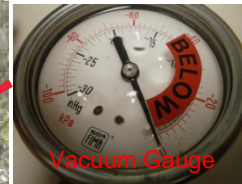
Positive Containment Check
