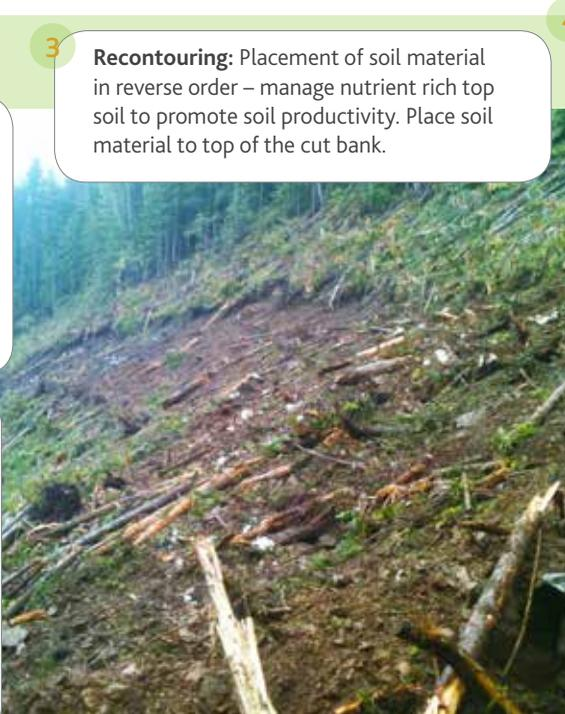
**3 Recontouring:** Placement of soil material in reverse order – manage nutrient rich top soil to promote soil productivity. Place soil material to top of the cut bank.
