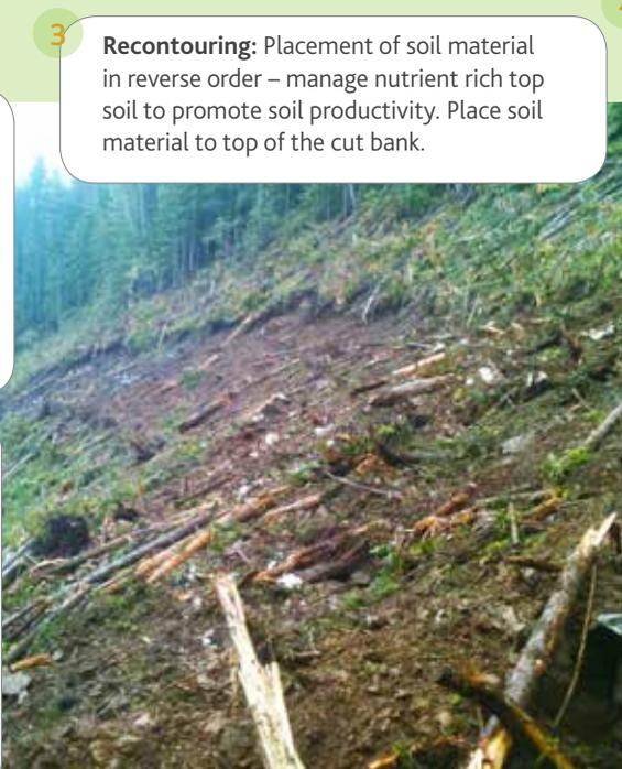
**3 Recontouring:** Placement of soil material in reverse order – manage nutrient rich top soil to promote soil productivity. Place soil material to top of the cut bank.
