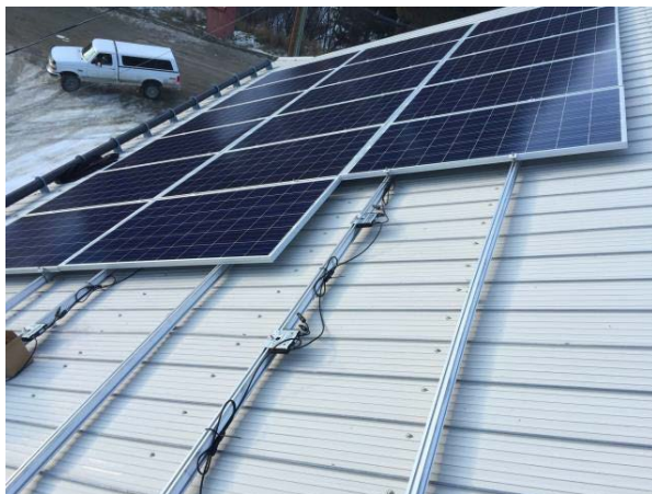
Community Building Installation
