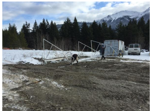
Transfer Station Installation
