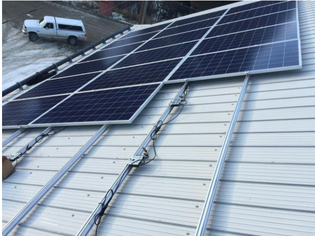
Community Building Installation
