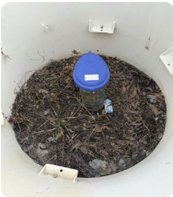
Figure 2. A well head for a deep water well. Calculating water demand and ensuring wells have adequate supply is crucial. If the well recharge rate is too low, cisterns will have to be incorporated into the design to ensure continual supply.
