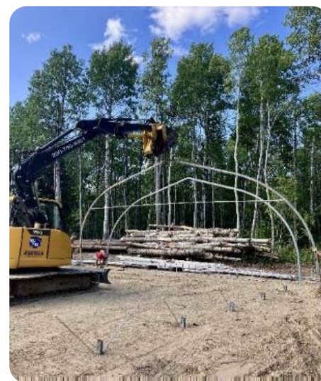
Figure 4. Using a compact excavator to assist with installing new 80 ft greenhouse
