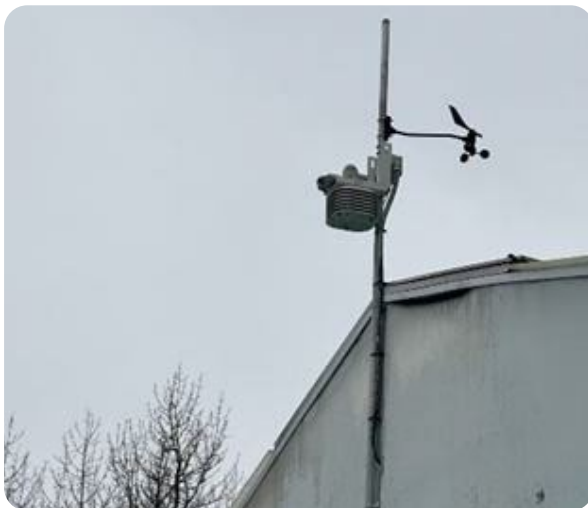
Figure 11. A weather station was installed on the greenhouse ridge. These systems can be used to control automation within the greenhouse.
