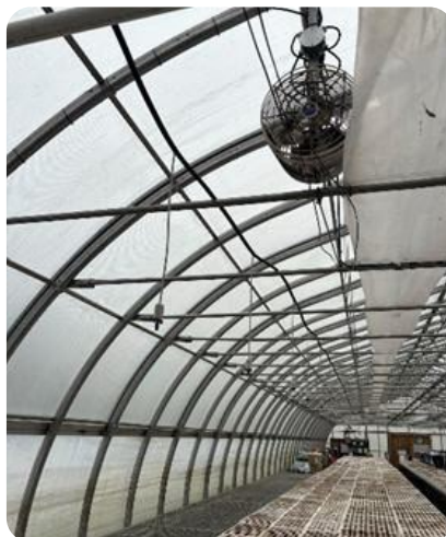
Figure 5. HAF fan provides air flow inside the greenhouse. This helps mix warm and cool air in the greenhouse and lowers the chance of fungal diseases.
