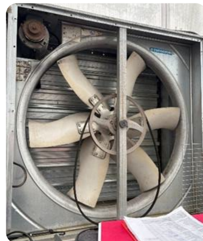
Figure 6. A large exhaust fan. These are important for growing in heated greenhouses during winter because they help control temperature and humidity without needing to open roof or wall vents.
