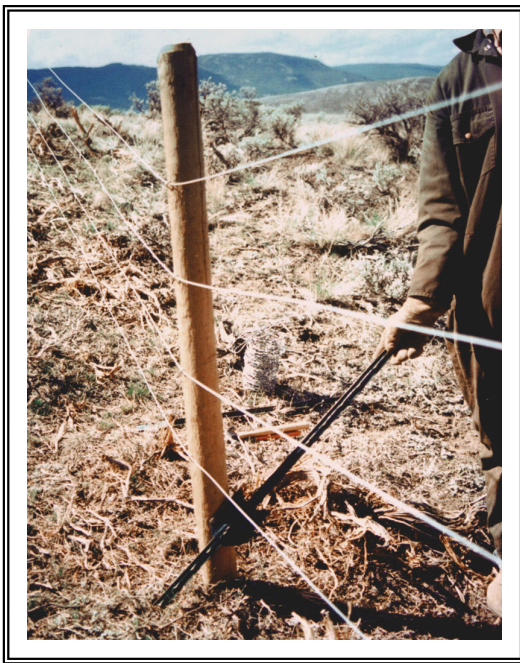
Figure 8 Footing a Dip Post
