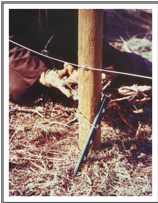
Figure 8 Footing a Dip Post
