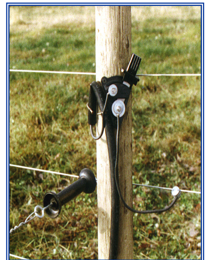
Figure 9 Typical Cutout Switch
