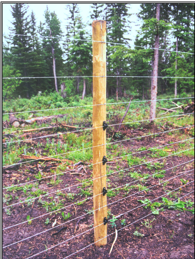
Figure 1 Typical Elk Line Fence Showing Line Post, Wire and Insulators
