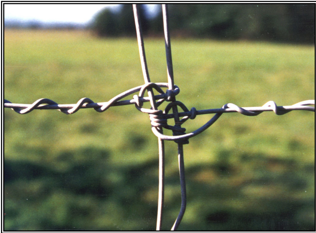
Figure 4 Splicing Woven Wire
