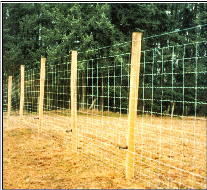
Figure 1 Typical Elk Exclusion Fence Using Woven Wire
