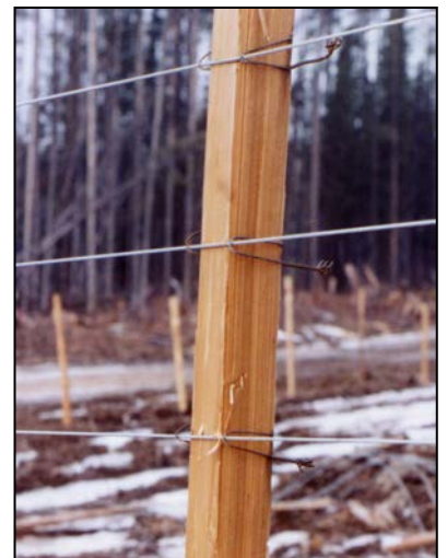
Wire-tied Wooden Dropper on HTSW
