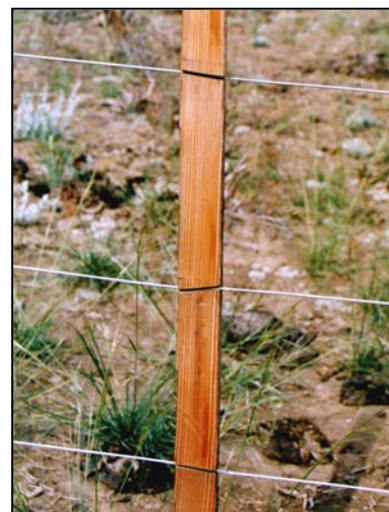
Angled Slot Dropper on HTSW
