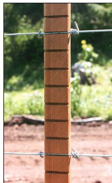
Horizontal Slot Dropper on HTSW
