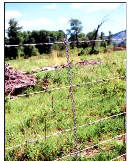
Metal Dropper on Barbed Wire
