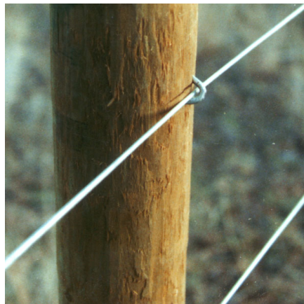
Figure 1 Loose Stapling of Fence Wire
