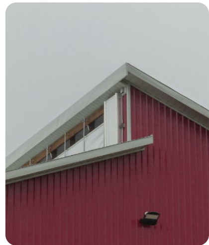
Figure 4. Offset ridge opening with adjustable curtain.
