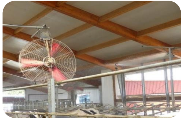
Figure 1. Sprinkler system with low pressure large droplet nozzles
