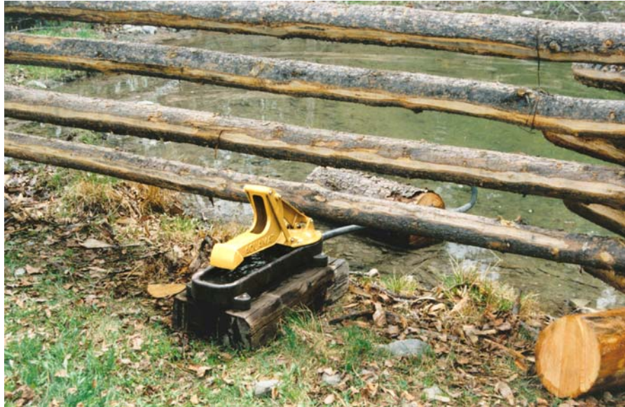
Figure 7 Rail Fencing at Nose Pump Location
