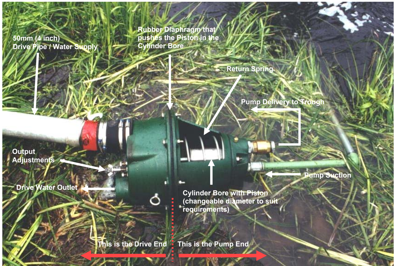
Figure 1 Glockemann 320 Oasis Pump Installed Along Watercourse (delivery line not shown)
