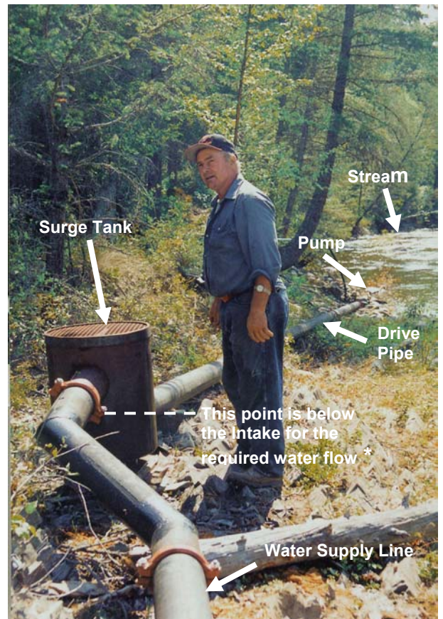
Figure 6 Surge Tank Setup
