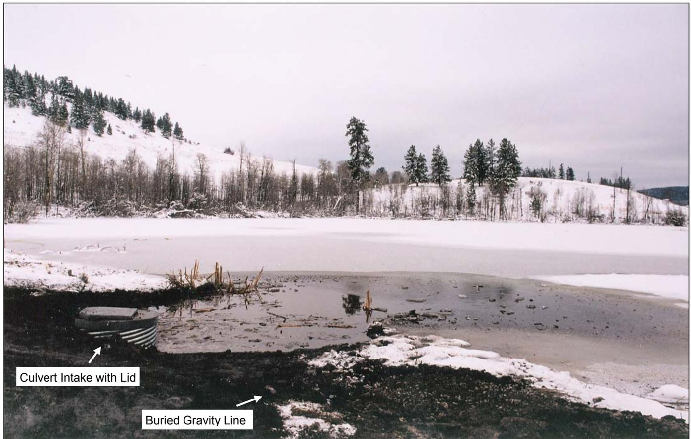
This grazing area water source is gravity fed to a livestock waterer 400 feet away. Note the culvert intake with lid.
