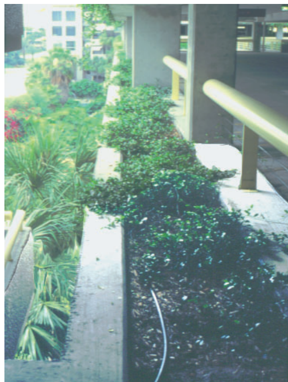
Figure 15.4 Planting Bed with a Single Lateral Line
