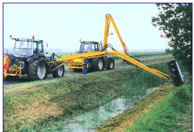
Figure 1 Mowing a Ditch From One Side
