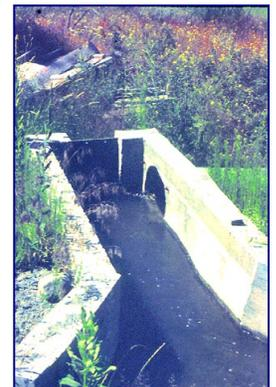
If concrete is used in the construction of the diversion structure, use prefab concrete wherever possible. If
