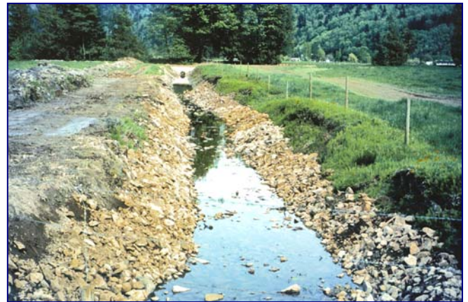
Figure 1 Riprap Placement on a Constructed Ditch
