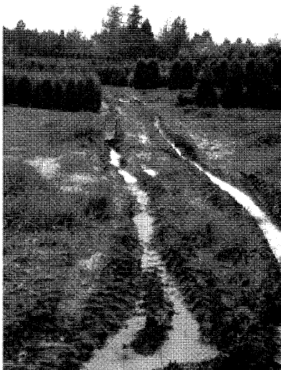
Figure 4.6 Compaction & Rutting – Indicators of Poor Drainage
