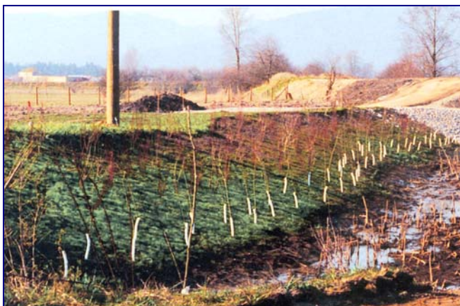
Figure 2 Live Staking
