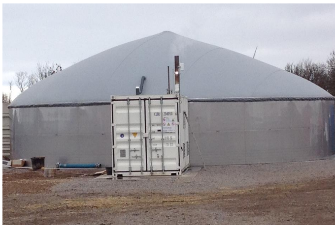
Example of Bioelectric modular biogas plant. Source www.bioelectric.be/en
