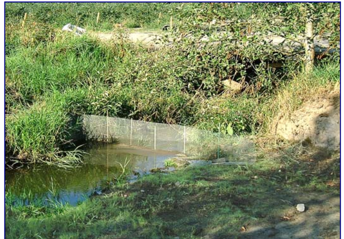
Figure 1 Sediment Trap with Temporary Silt Fence During Cleaning
