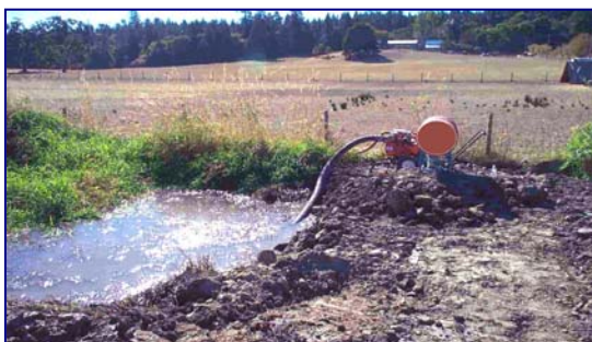
Figure 9 Pumping Over Temporary Clay Dam
