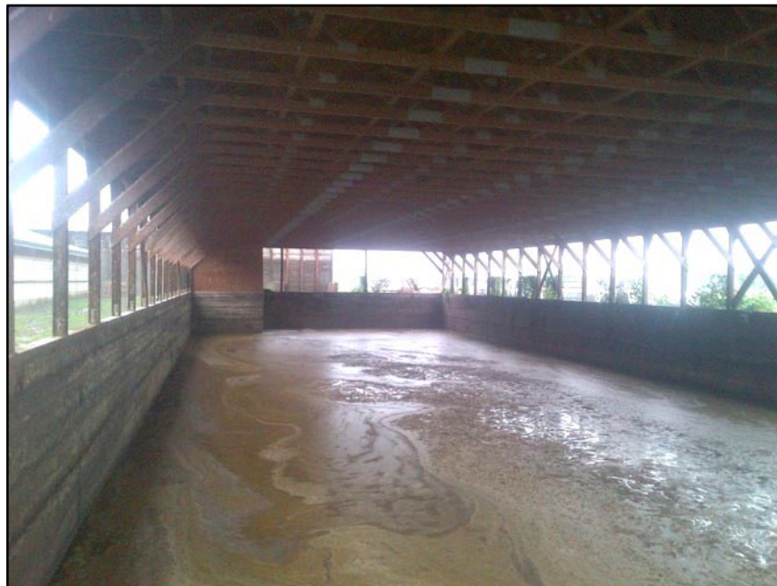
Figure 4: Example of liquid manure storage improvement including manure storage expansion and roof.
