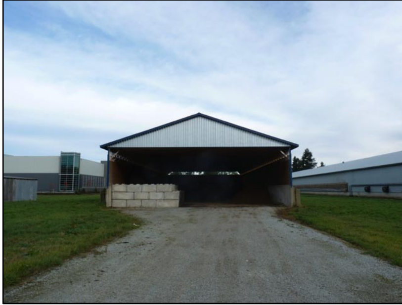
Figure 5: Example of solid manure storage improvement including manure storage expansion and roof.
