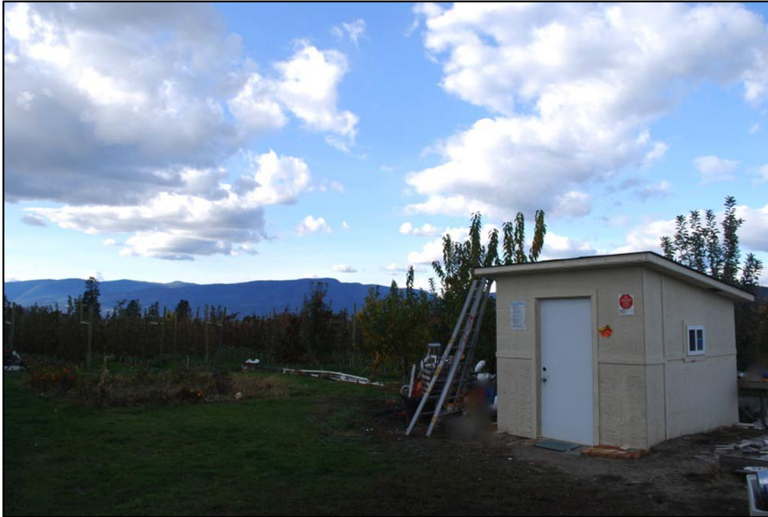
Figure 15: Pesticide shed funded through the BMP programs
