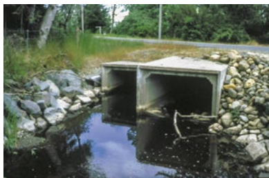
A box culvert that provides fish passage
