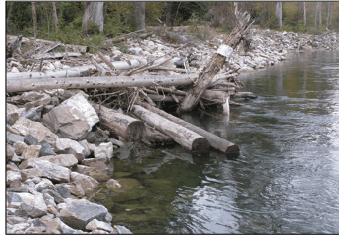
Bio-engineering river bank restoration.
