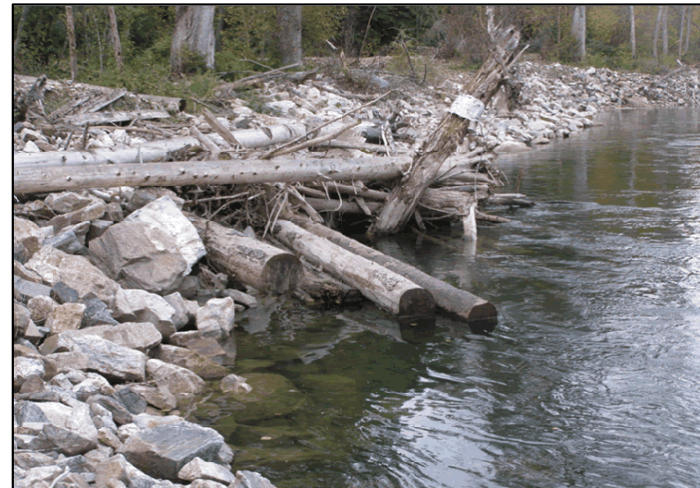
Bio-engineering river bank restoration.
