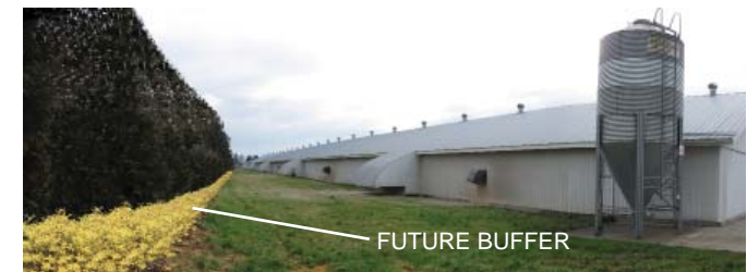
View of future vegetative buffer
