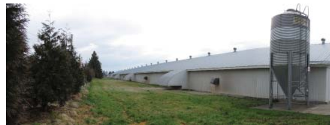
View of existing site
