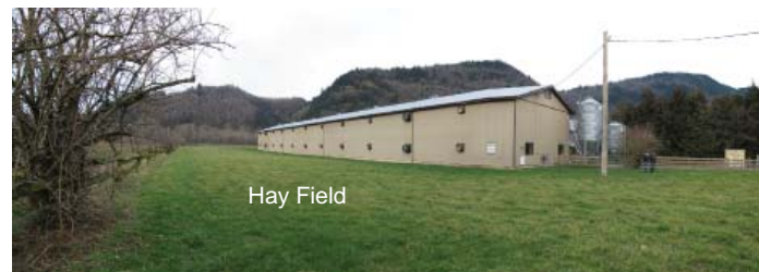
View of existing site
