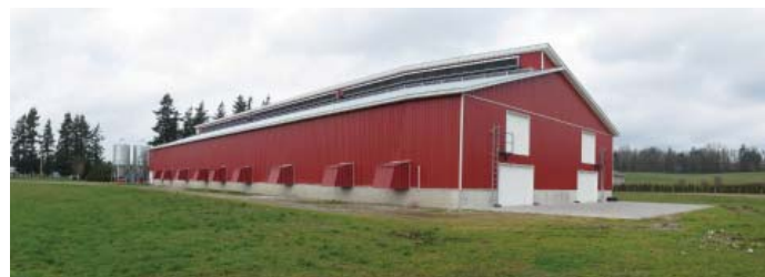
View of existing site
