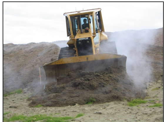
Photograph 23: Spreading pulp and paper residuals with a dozer
