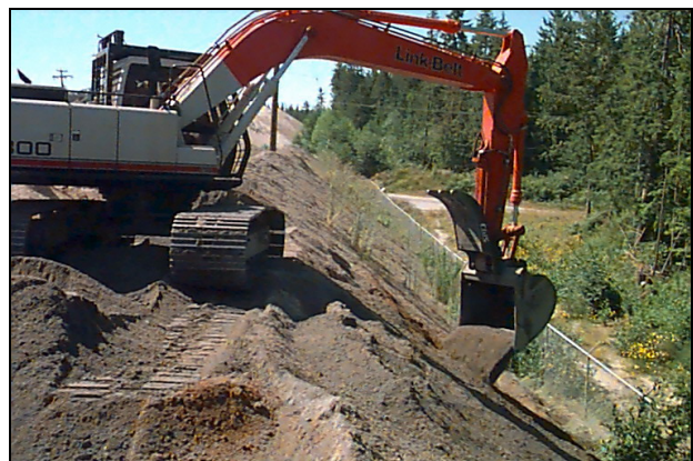
Photograph 32: Excavator casting a pulp and paper residual and sand mix over a slope
