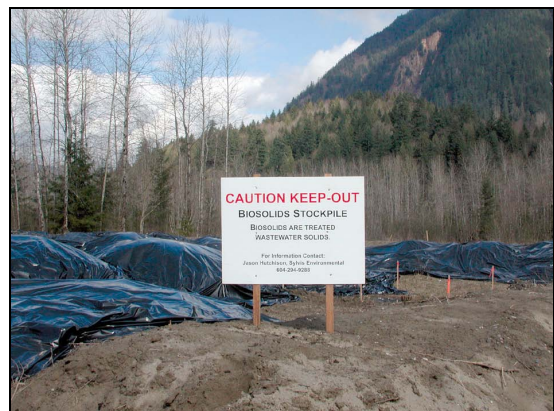
Photograph 20: Signage posted on an earth berm surrounding a covered biosolids stockpile
