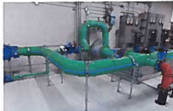
Polypropylene pressure piping in commercial plumbing application.
