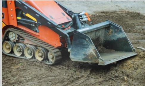
A report prepared by Sage Policy Group explains in depth several of the major concerns in the construction industry in BC.
