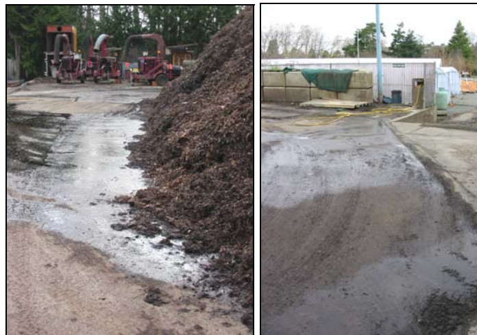
Figure 3 Leachate contained by an asphalt berm and directed to a collection sump.
