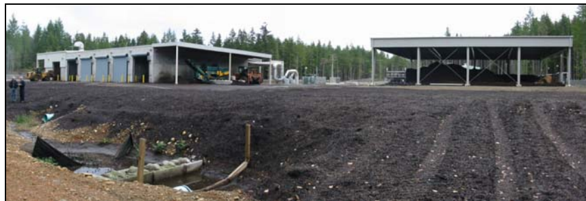
Figure 4 The Site H invessel composting facility. To the left is the compost building housing the mixing, composting bins and screening facilities. To the right is the curing building. A leachate collection pond is shown in the lower left of the photo.
