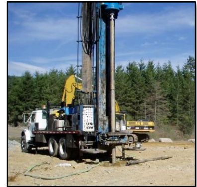
Figure 1 - Vibrasonic drill rig.
