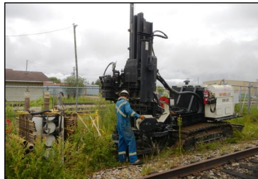
Figure 8. Direct push track-mounted drilling rig.
