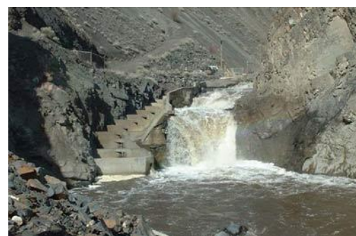
Repaired fishway (photo: MFLNRORD).
