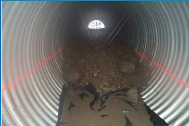
Substrate Installation
