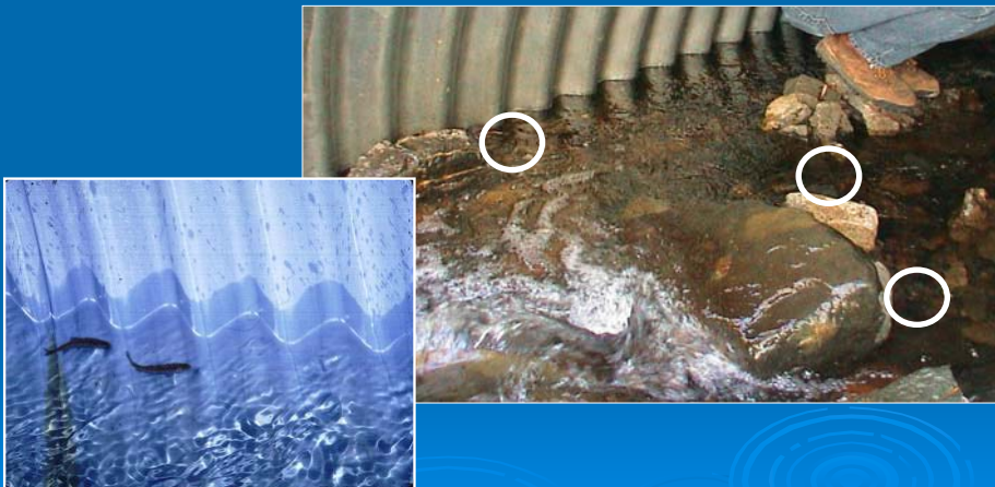
Roughness reduces velocity and creates shadows
