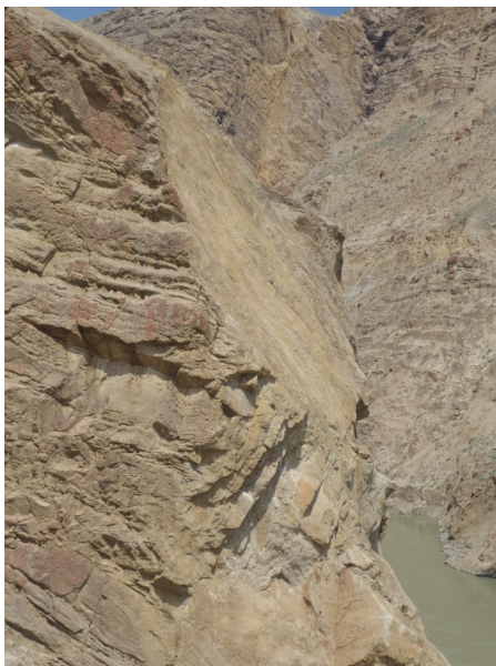
The height of the rockface is approximately 120 metres.
