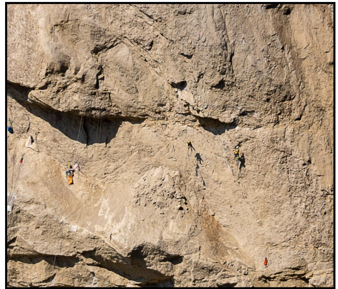
Scalers on the rockface above the landslide.
