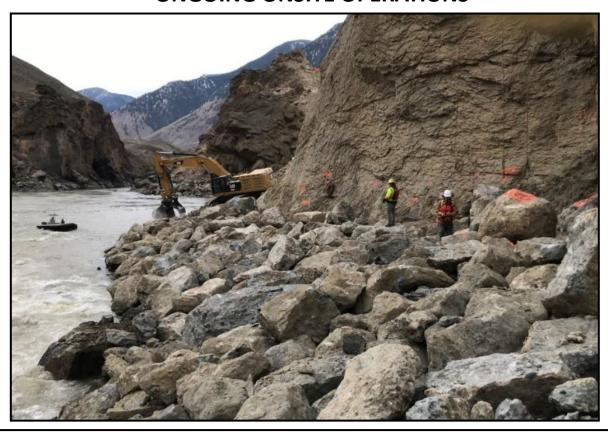
**PICTURED:** Crews putting the final touches on the "nature-like" fishway, which was completed last week on the west side of the slide site
