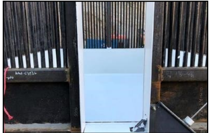
PICTURED: DFO staff painted parts of the hopper with white marine paint to protect fish from abrasion from the metal surface and to increase visibility for counting the salmon.
