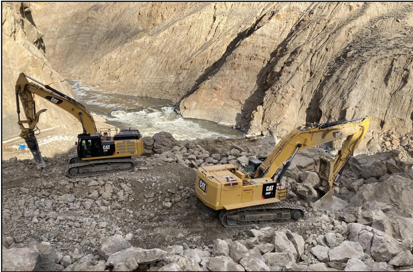
**ABOVE:** Equipment sorting shot rock and riprap material at the Razorback. This material will be used to create temporary access and construct the embankment for the permanent fishway.
