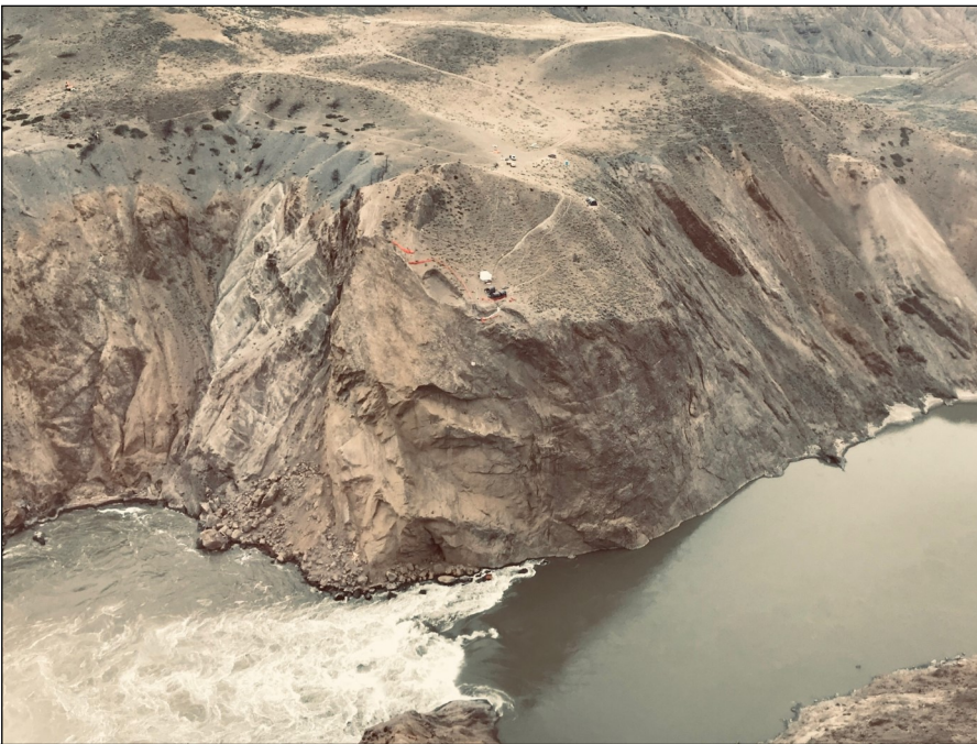
Aerial photo of the Big Bar Landslide on Sept 19 showing high water levels.
