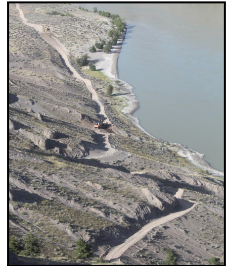
Road construction progress.
