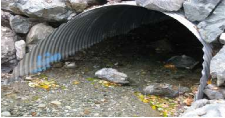
Figure 1: Properly embedded culvert. Streambed is continuous and 40% of culvert diameter.
